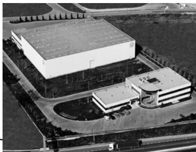
Logistics Center in Parets (Spain)
